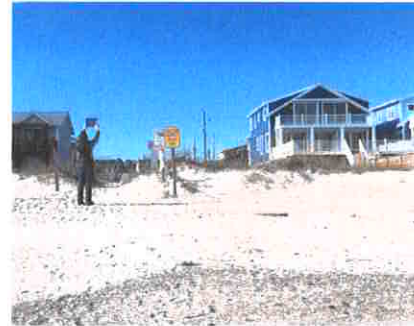
Photo 2: Showing location of underground storm drain.
