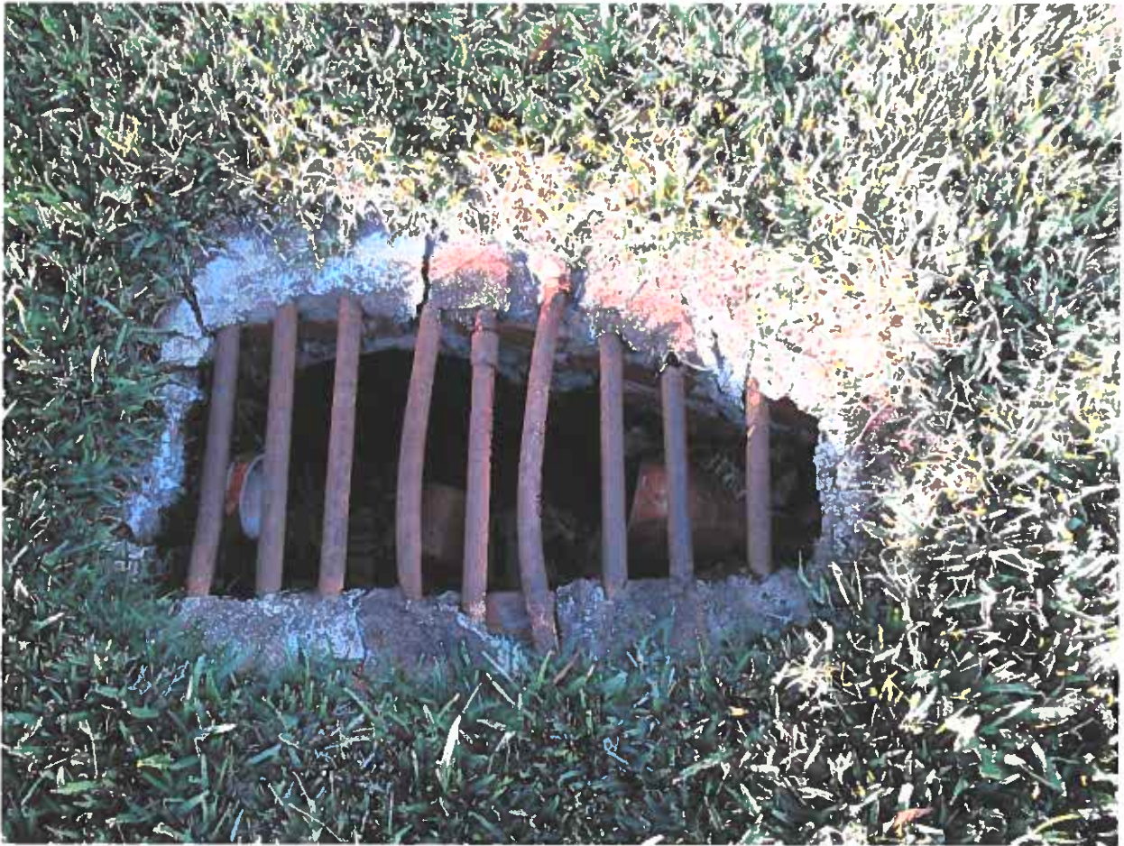
Figure N: "Homemade" Yard Inlet
