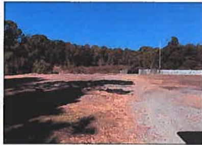
Existing conditions looking north to Spot Lane
