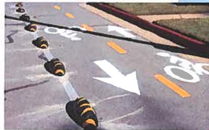
Example of an "armadillo buffer" being used to buffer on-street space for bicycling.
