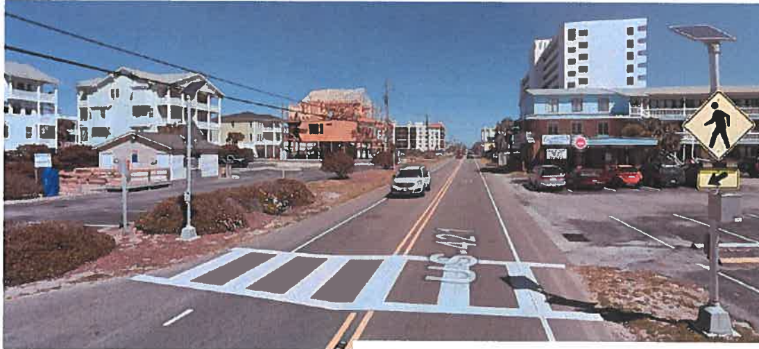
Example of the recommended flashing beacons for beach access points (in Carolina Beach)
