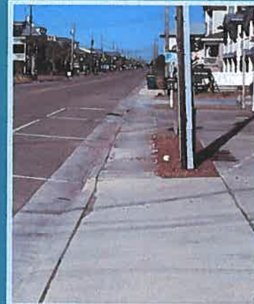
Existing conditions along Fort Fisher Blvd on the east side of the street (looking north).
