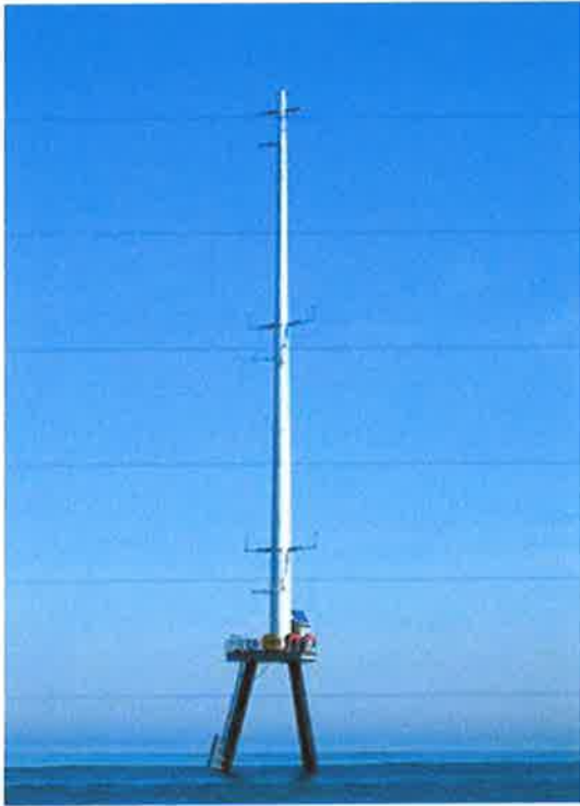
Figure 3-5 Example of Monopole-mast Meteorological Tower
