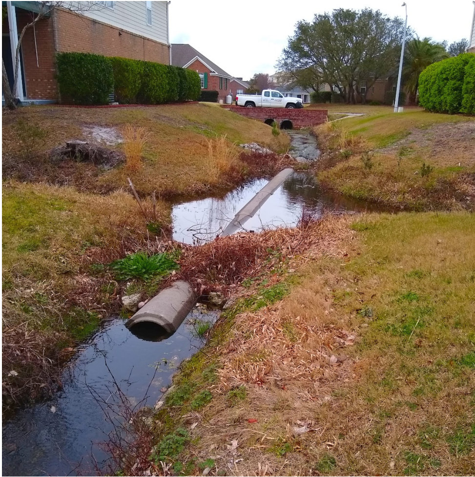
Figure L: 18" Pipe Within Ditch Connecting the Ponds
