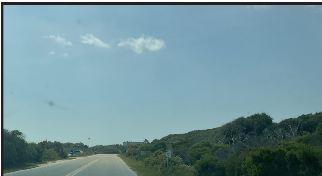
29 Existing Road Next to Wetlands
